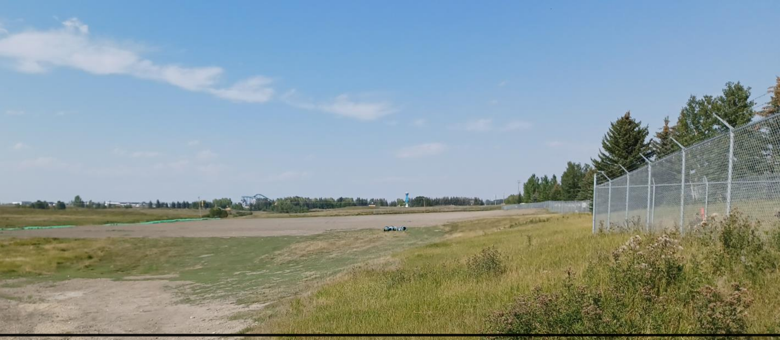
Elbow Valley – Lagoon Reclamation
