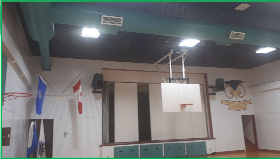
Crossfield Elementary Painting, Flooring, LED Lighting
